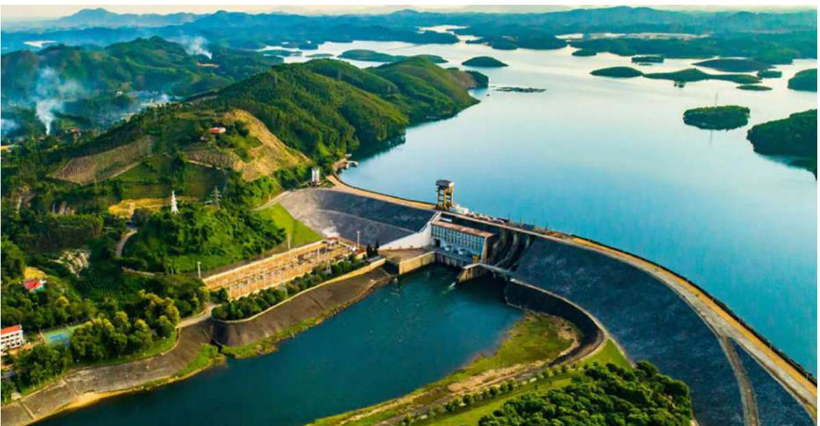
Source: Thac Ba Hydropower Plant 2014, Ree Corporation
